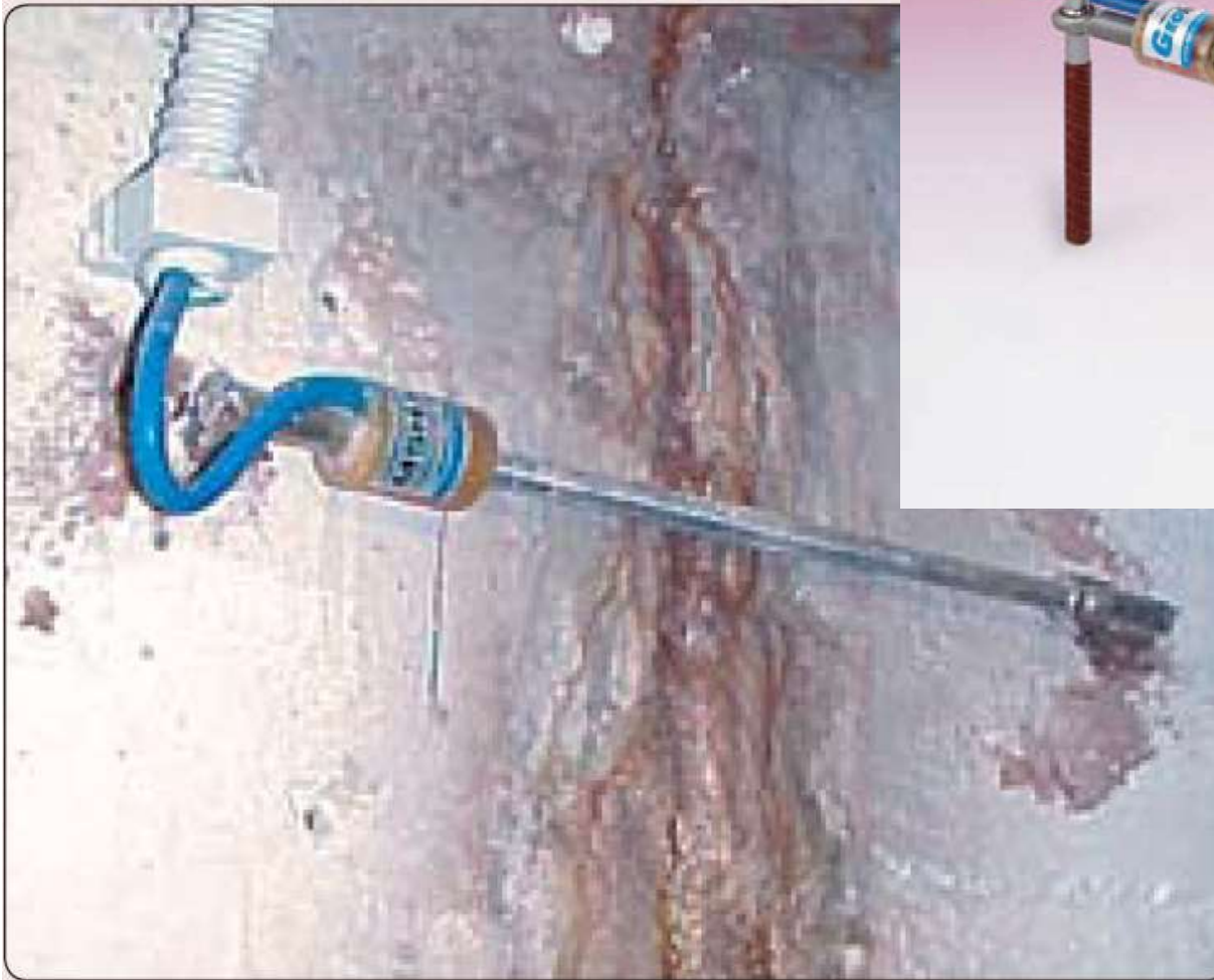
● Model 4420 Crackmeter installation.
