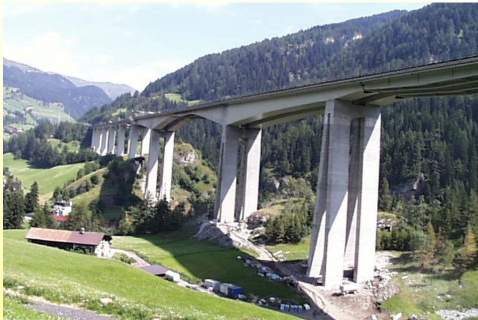
Colle d'Isarco bridge. Brennero highway, Italy
